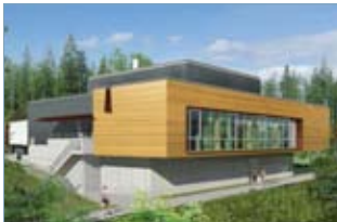
Architectural Rendering of UNBC Gasification Facility
