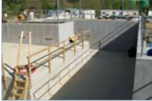
ORNL Gasification System Construction
