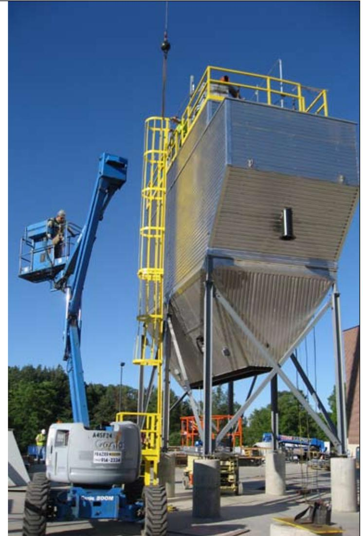
Electrostatic Precipitator (ESP)
