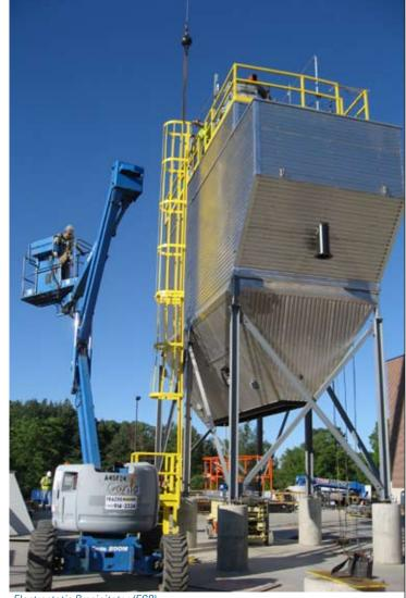
Electrostatic Precipitator (ESP)
