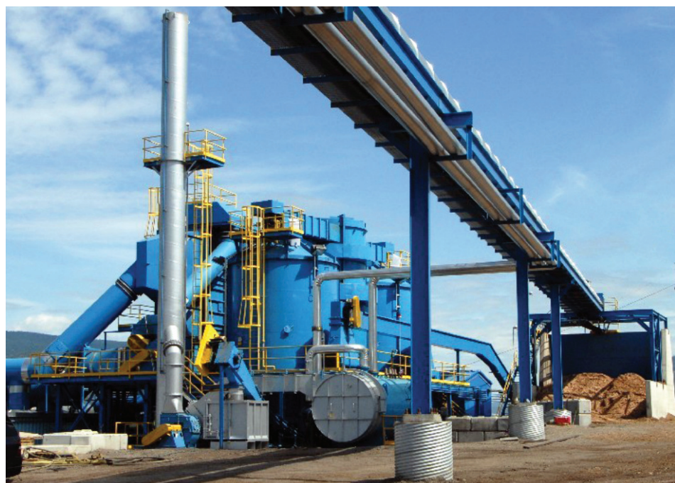
Nexterra's gasification project for Tolko Industries in Kamloops, B.C.
